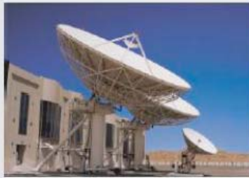
Earth Station in Sharjah / UAE
