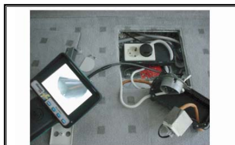
Visually Checking Underfloor Ducts
