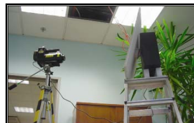
X-Raying Wall Ceiling Cables
